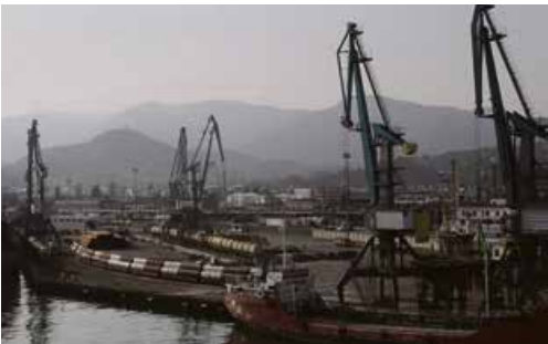
Harbour facilities to be improved and extended
